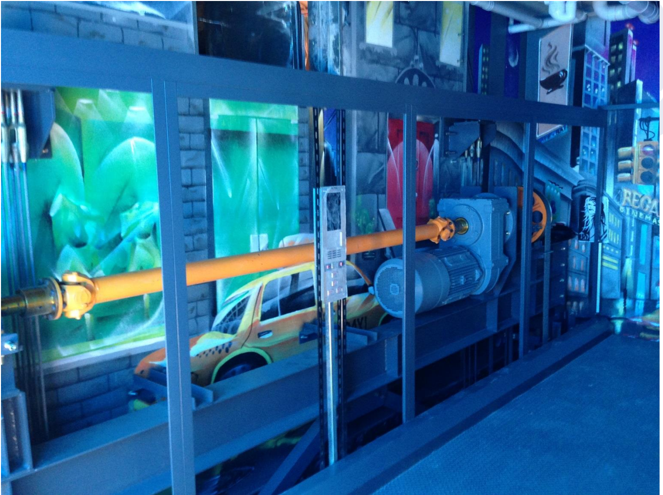
(Figure 6; 45 Maxwell St, Newfarm. Main lifting motoring and driving mechanism)
