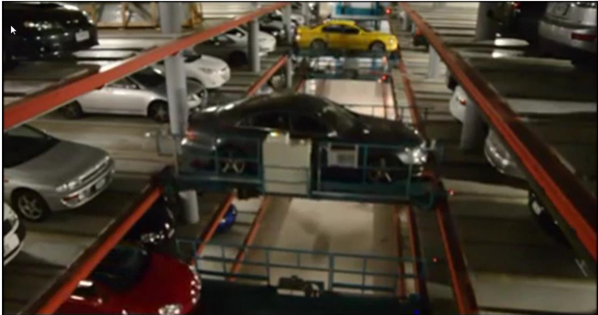
(Figure 9 ; Fully Automates Car picker installed by Hercules in Newzealand providing 176 spaces)
